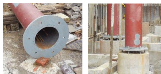
Figure 4: Base plate for CFST column
