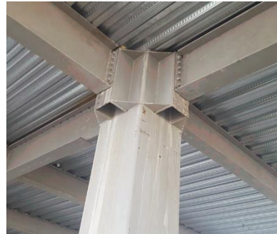
Figure 8: CFST column connection at floor level
