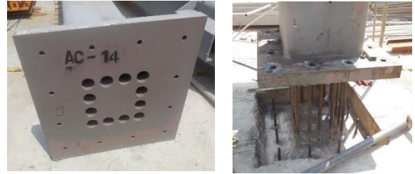
Figure 7: Base plate for CFST column
