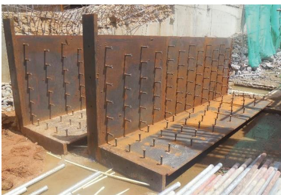
Figure 10: Shear connectors for steel jacketing
