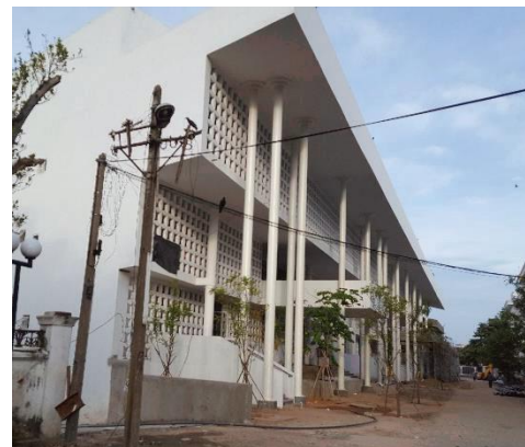
Figure 3(b): CFST slender columns – building 2
