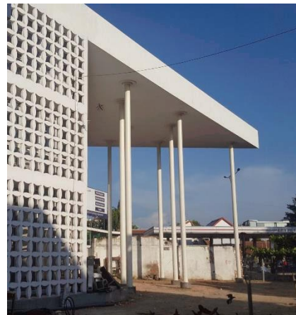
Figure 3(a): CFST slender columns – building 1
