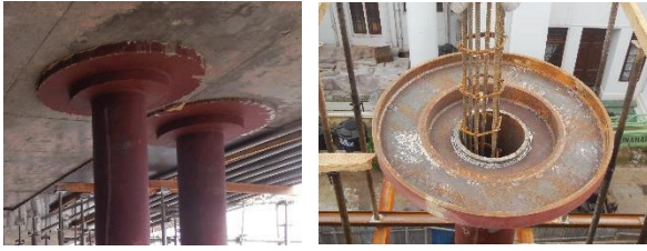
Figure 5: CFST column head detail at flat slab
