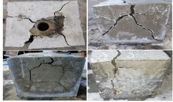
Figure 6: Cracks specimens with encased concrete
