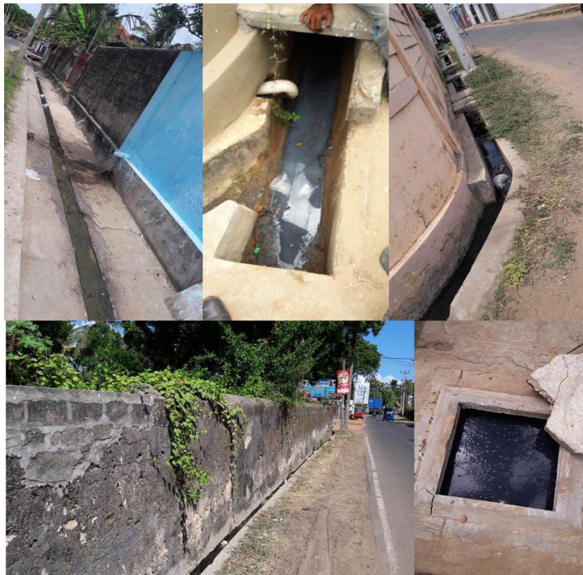
Figure 3: Open surface drain system in Jaffna city that increases ground water pollution and provide sites for preimaginal development of mosquito vectors.
